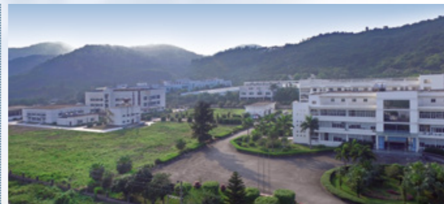
Oversea plant 海外工厂 Zhuhai Jinwan District - China
